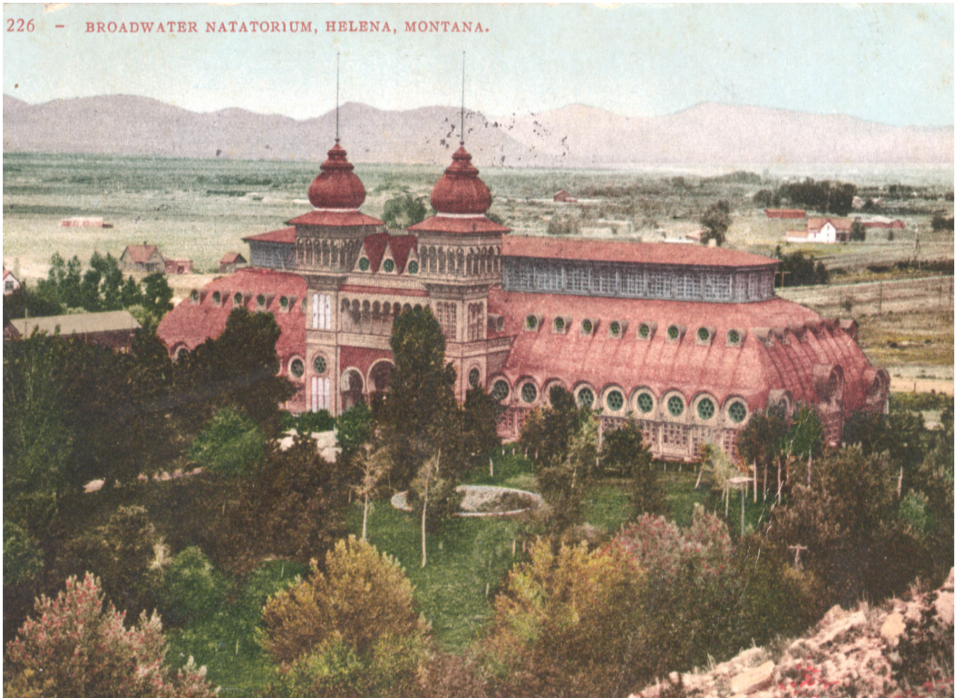
Exterior of Broadwater Natatorium near Helena, circa 1889.
